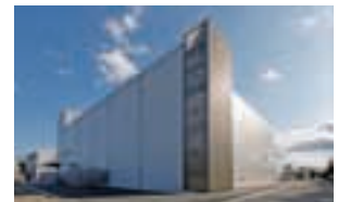
A Pharmaceutical Raw Material Building
