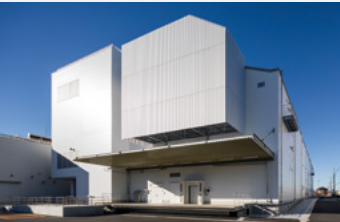
DS manufacturing building, “HB7”
