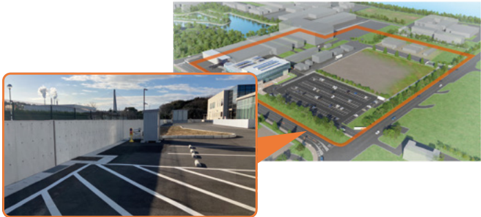
Installation of tidal embankment (Ube Plant)
